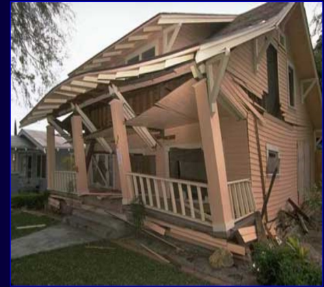
Residential damage caused by the 1994 earthquake in Northridge, California. Photo courtesy FEMA
