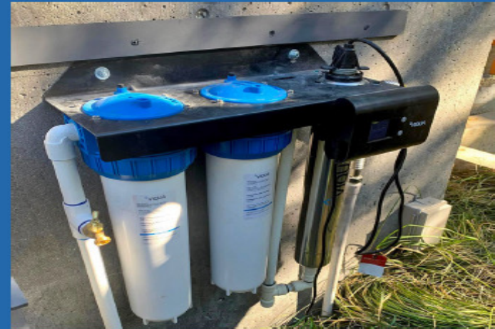
Filtration + UV sterilization bank
