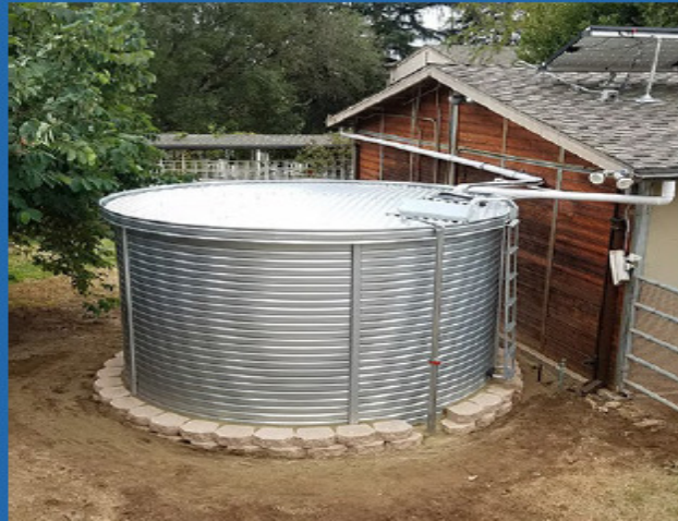
Large above ground tanks
