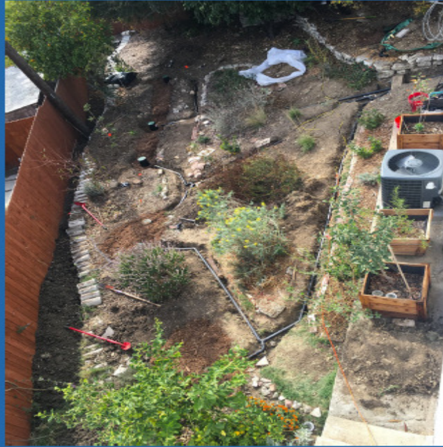
Branched drain system before, during and after installation
